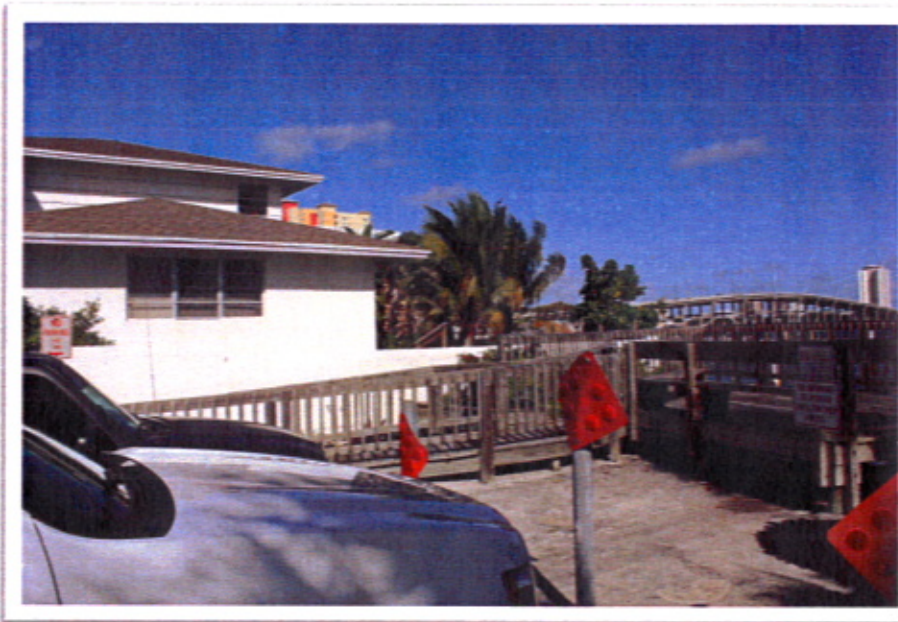
Figure 2 256 E 22nd Ct with Adjacent "Observation Deck"
