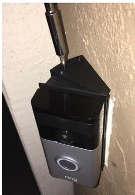
14. Screw in the screws at the top and bottom of the front part of the doorbell.
