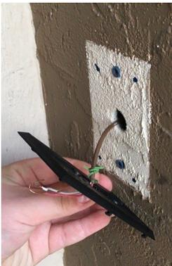
1. Take the backing of the Ring device and place it on the wall where your doorbell was and mark the screw holes with a pen or marker on the wall behind the plate.
